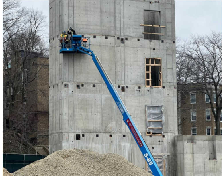
Welding Clips at Core C - in preparation for Steel erection start on 4/4/22. (Photo Below)
